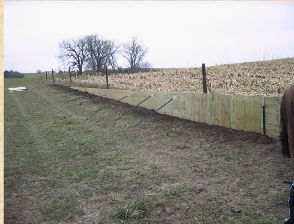
Completed 3 foot plywood wall, November 2009. (Took 1 day to complete with 6 people)
