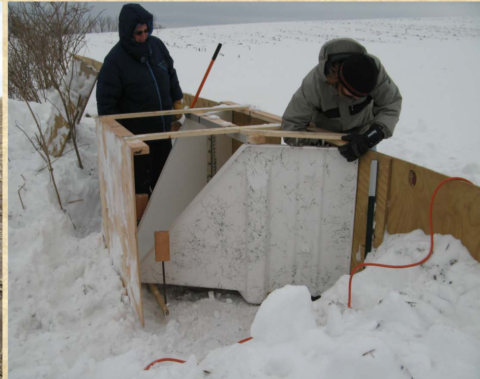
Installing H-flume into position at the lowest point on the field edge, January 2010.
