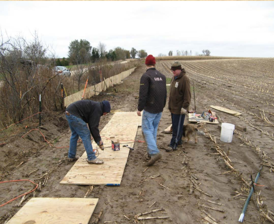
Constructing the plywood barrier for edge-of-field monitoring, October 2009.
